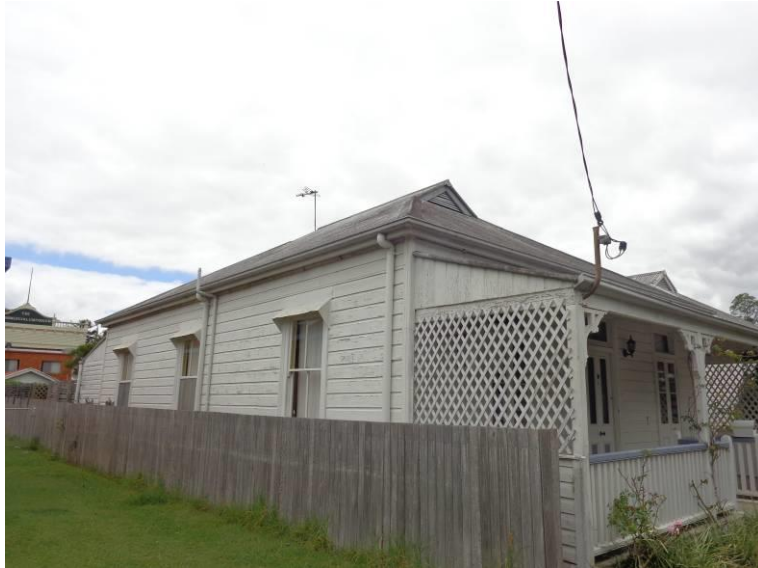
9 William Street proximity to boundary.
