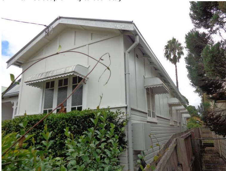
21 William Street proximity to boundary.
